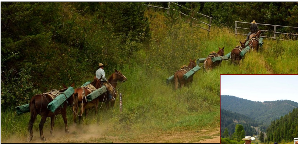
BCH members wrap timbers in canvas, load the timbers onto metal pack frames, put the pack strings together and head out to the bridge site.
